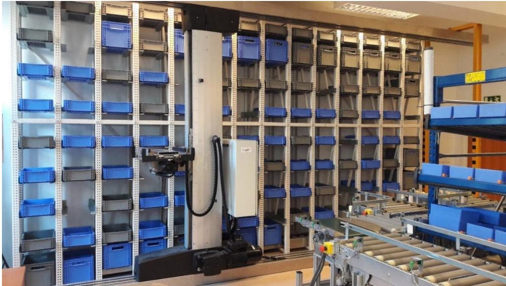
Figure 5. The storage system with the automated racking machine, together with the unloading segment of the rolling conveyor track (Source: created by the authors)
