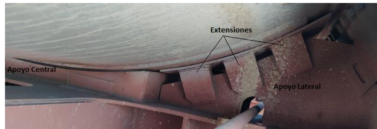
Figure 2.6 Lower supports at the ends of the rail-tank. Source: (author)
